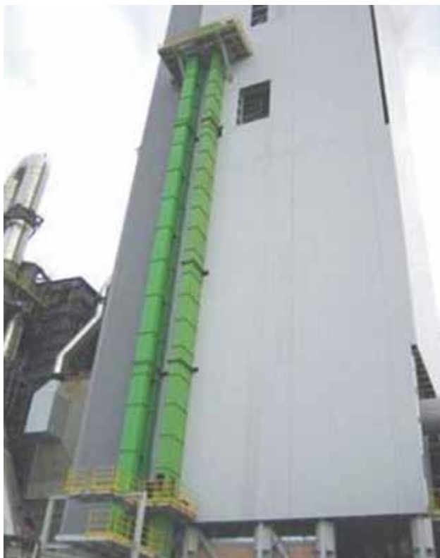
Figure 2. High capacity bucket elevator for RDF and other alternative fuels
